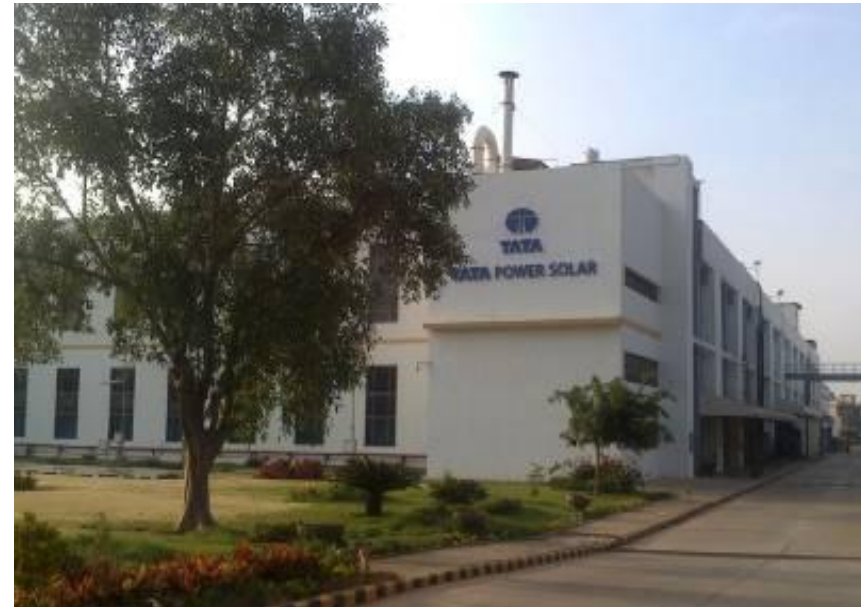
Tata Power Solar module manufacturing facility
